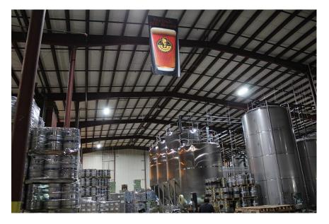
GreenTech carefully assessed the lighting needs and energy usage of the brewery and custom-designed a lighting plan. The LED lighting upgrade in the brewery brought significant energy savings for the 48,000-square foot facility. After legacy high bays and T12 fluorescents were replaced with energy-efficient LED fixtures, **the brewery experienced a 68 percent reduction in annual operational costs.** A summary of benefits is as follows:
